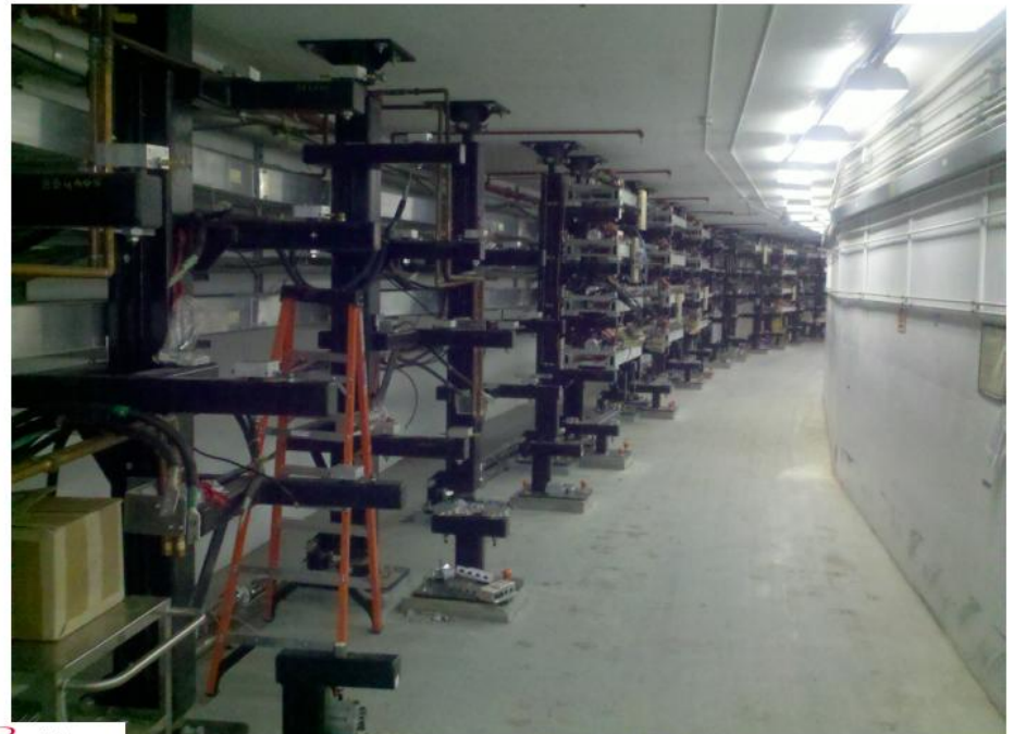
Dipoles all removed!!!! West Arc circa July 2011
